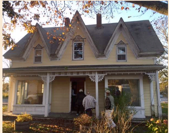
OHS Board members recently toured the Bassett house on Cranberry Highway.
