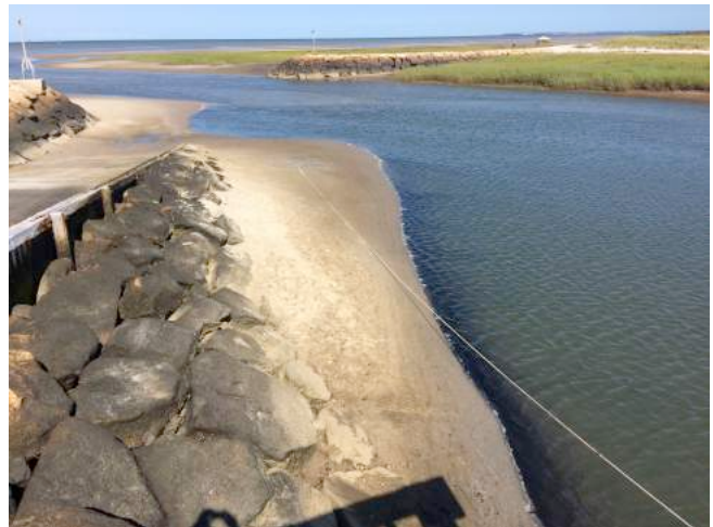
Spare anchor line is tied to buried anchor for extra safety.
